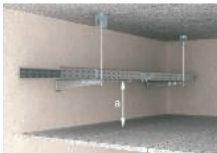
Distance to false ceiling for cable tray, type SKS: see mounting parameters for distance a.
