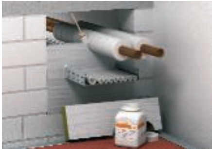
Coat the full length of the path insulation with the paint (dry layer thickness at least 1 mm).
