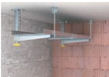
One-layer cable-specific support construction made of EKS cable tray with U suspended support, bracket mounted on one side.
