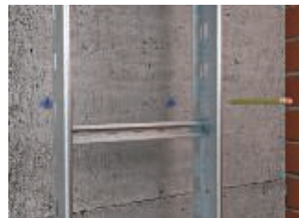
Transfer the position of the holes drilled in the vertical ladder to the wall.
