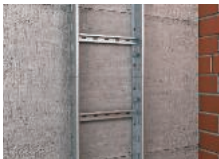
Standard support construction made of vertical ladder L 6... VS. The joint is mounted without connectors.
