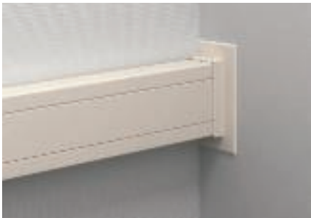
Mount the duct lid and wall connection panel.
