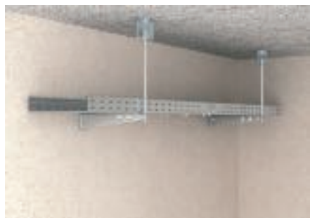
Routing system for ceiling mounting of the cable tray of widths 200 mm to 600 mm.
