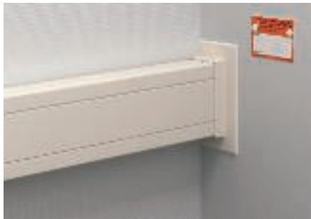
Filling out of the wall plate and fastening next to the insulation. Filling out of the declaration of agreement and handing over to the client.
