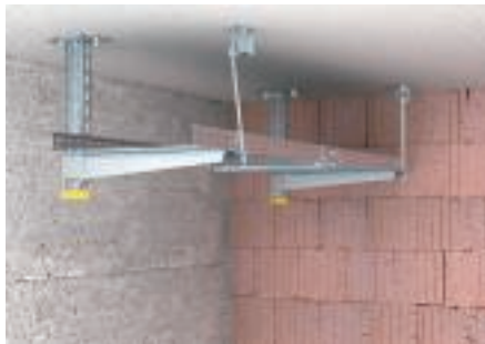
Mounting of threaded rod
