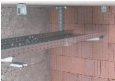
Mounting of connection component
