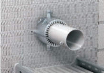
Mounting of the threaded rods (M6 or M8) and fastening of the pipe seal(s).
