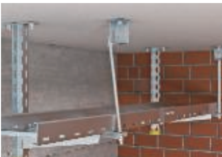
Mounting of threaded rod
