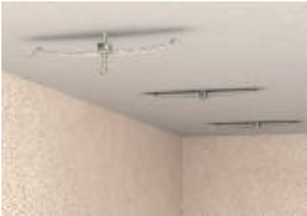
Push the fire protection bolt tie through the fastening hole of the pressure clips and fix in the drill hole.
