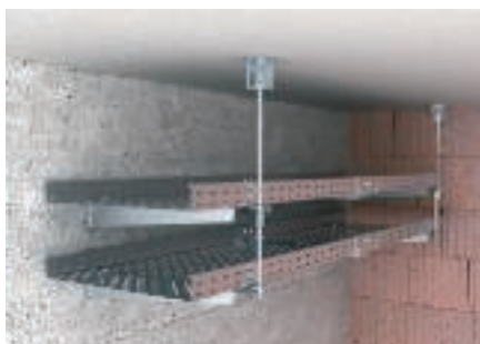
Two-layer cable-specific support construction for wall mounting with EKS cable trays and threaded rod locking vertically to the ceiling.
