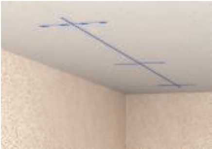
Draw on the exact position of the drill holes for the pressure clips using a chalk mark.
