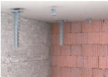
Support and clamp mounting
