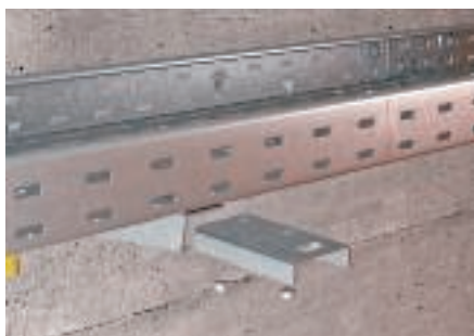
Mounting of connection component
