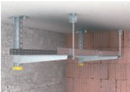
Locking the threaded rod
