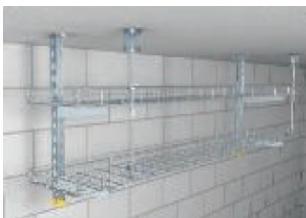
One and two-layer routing of GR-Magic mesh cable trays.
