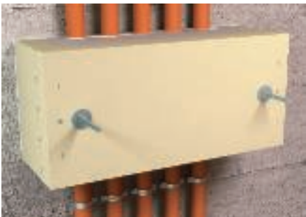
Strain relief with OBO ZSE 90. Approved for all cable types, function maintenance class E 30 and E 90.
