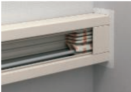
Complete closing of the duct interior using three different bag sizes. Fill any spaces, in particular the spandrels between the cables.
