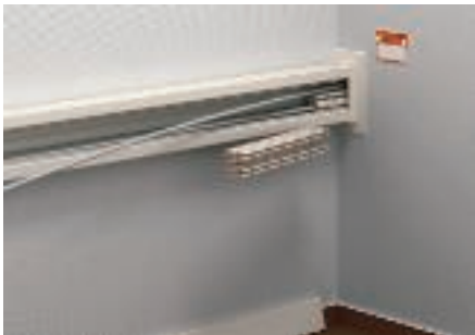
Remove of the duct lid next to the insulation. Remove of bags from the insulation After cable insulation, close the duct interior as on first construction.
