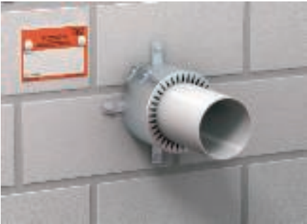
Completion by filling out and mounting the identification plate and handover of the completed declaration of agreement to the client.
