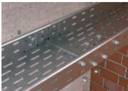
Straight and floor connector mounting
