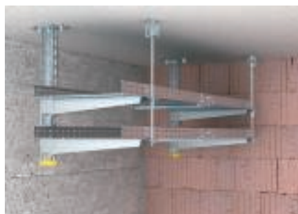
Two-layer cable-specific support construction made of EKS cable trays with U suspended support, bracket mounted on one side.
