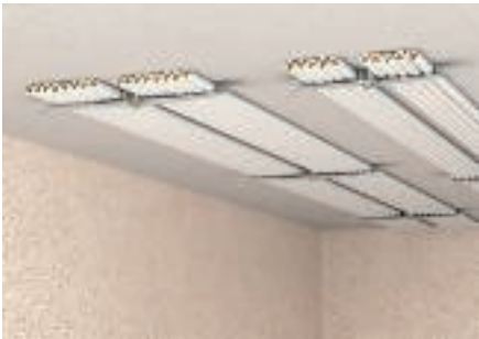
Push the fire protection bolt tie through the fastening hole of the pressure clips and fix in the drill hole.
