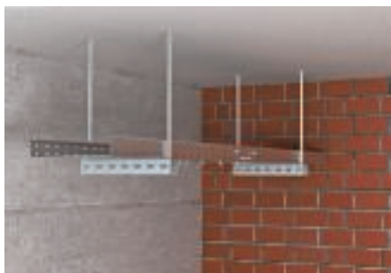
One-layer standard support construction made of an SKS cable tray and threaded rod suspension on both sides and cross-section, type US 3/....
