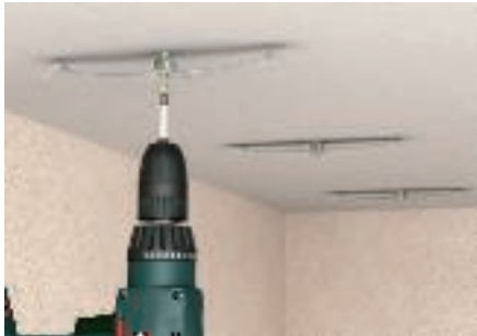
Turning of the bolt tie into the drill hole. Turning in can take place using a rechargeable or ratchet screwdriver, or also by hand.
