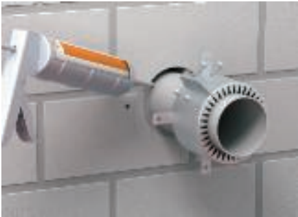
Before mounting the pipe seal, close the ring gap with fire protection filler or mineral mortar.
