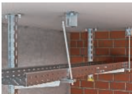
Mounting of threaded rod
