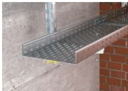
Mounting of the cable tray on brackets
