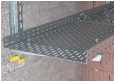
Mounting of the cable tray
