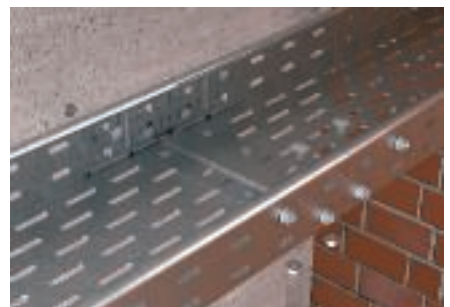
Straight and floor connector mounting
