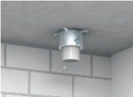
The round, screwed-on CRM is also fastened from below using metal anchors.
