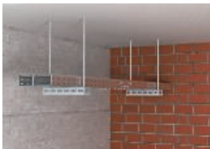
One-layer standard support construction made of two SKS cable trays and threaded rod suspension on both sides and cross-section, type US 5/....
