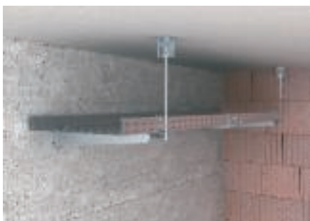
One-layer cable-specific support construction for wall mounting with EKS cable tray and threaded rod locking vertically to the ceiling.
