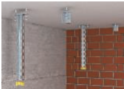
Support and clamp mounting
